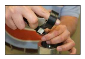
10. To ensure the connection stays together, put a few wraps of electrical tape around the connector.
